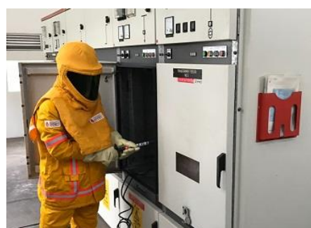
Maintenance of 22kV HT Switchgears
