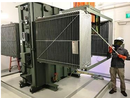
Maintenance of High Tension Transformers
