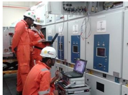
Testing of Protection Relays at 22kV HT Switchgears
