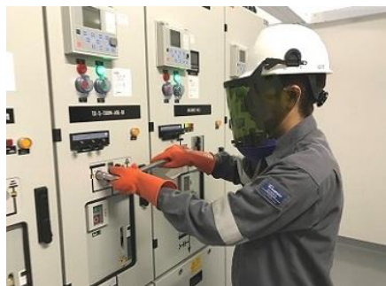
LEW carrying out switching at HT Gas Insulated Switchgears
