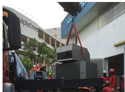
Installation of Switchboards / Transformers
